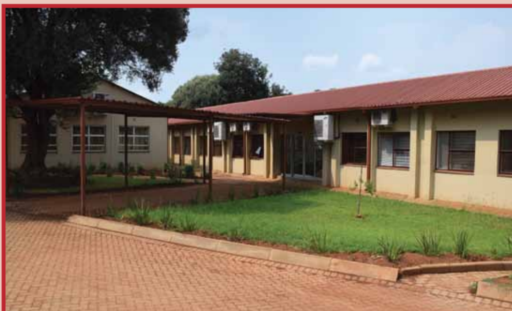
The newly refurbished Old Nurses' Home (Tharabollo) premises
